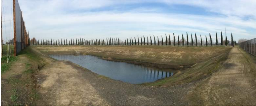
The River Bluff Detention Basin receives stormwater from the northern portion of the City. This large basin is very deep, which allows the stormwater to flow by gravity into the basin, thereby preventing the need for a stormwater pump station.
