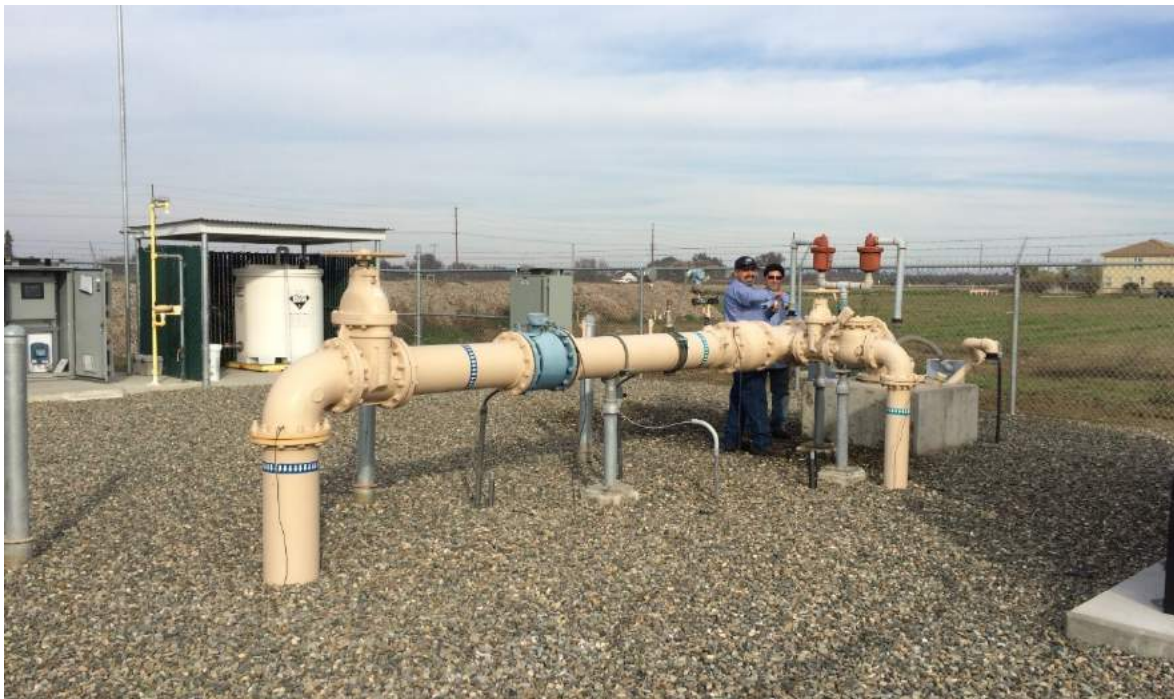
Well 38 has a capacity of 1,500 gpm. City staff performs routine water quality monitoring of the water quality and maintenance of the water system.
