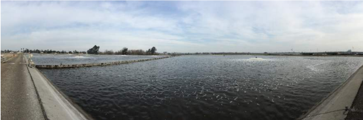
The WWTP aerated ponds treat the organic wastes from the wastewater. These ponds are lined with concrete to prevent the untreated wastewater from reaching the groundwater.
